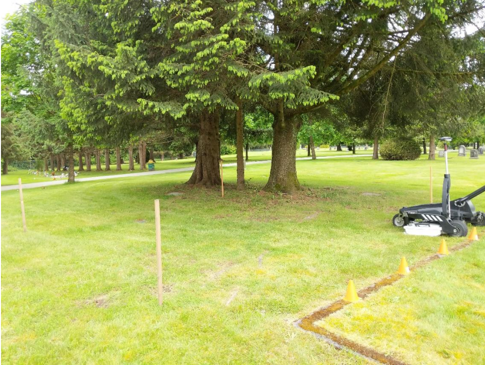
Photo 1: set-up of grid data collection. Concrete curb used for position reference. Start line approx. 60cm (2ft) parallel to curb.
