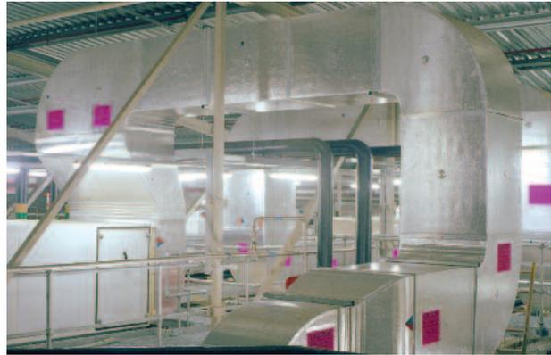
A key factor in the difference shown is in the cost of labor man-hours. The construction, installation and insulation activity of the sheet steel ductwork system, accounted for 714.75 hours. In contrast, the fabrication and installation of ductwork from The *Kingspan KoolDuct*<sup>®</sup> System, only required 513.75 hours – providing a labor man-hour saving of 28%.
