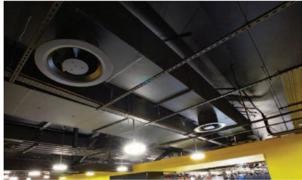
Ductwork fabricated from The *Kingspan KoolDuct®* System was the first premium performance pre-insulated ductwork in the world to be UL Listed as a Class 1 Air Duct, to Standard for Safety UL 181 (Underwriters Laboratories: Factory Made Air Ducts & Air Connectors), when fabricated to a specification clearly defined by UL.
