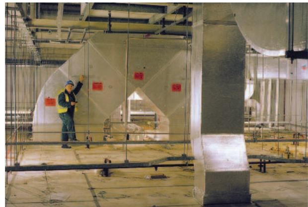
In the case of insulated HVAC ductwork, saving energy, by specifying the best ductwork air-leakage and heat loss / gain standards possible, is the most environmentally sustainable action to take when specifying ductwork and its insulation, since it is operational energy use that creates the vast majority of operational environmental impact.
