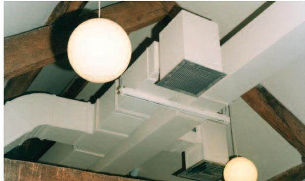
In addition, ductwork fabricated from The *Kingspan KoolDuct®* System can reduce air-leakage rates to a fraction of those typical of rectangular sheet metal ductwork. This cutting edge System thus offers the triple benefits of cutting energy use, cutting operational carbon dioxide (CO<sub>2</sub>) emissions and cutting costs.
