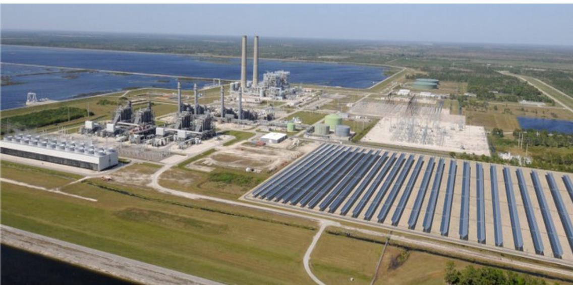
Rendering of Florida Power and Light's Martin Next Generation Solar Energy Center, a hybrid natural gas-solar plant in Indiantown, FL. The mirrors provide 75 megawatts of thermal solar power.
