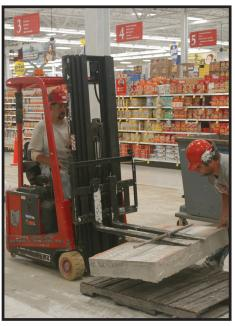
Ohio Concrete uses Electric Fork Trucks to remove concrete indoors.
