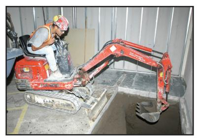
Ohio Concrete has a fleet of Electric Excavators that fit through a 34" doorway, yet will dig to a depth of 5 feet with no diesel fumes and no noise.
