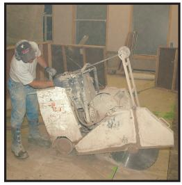
Ohio Concrete uses Fume-Free Electric Saws for inside work. Electric Saws reduce noise and the risk of carbon monoxide poisoning.
