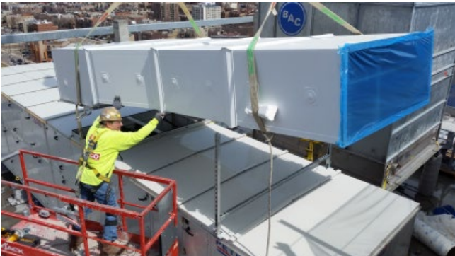
Flange is not a lifting point. Cradle ductwork with appropriate lifting straps.
