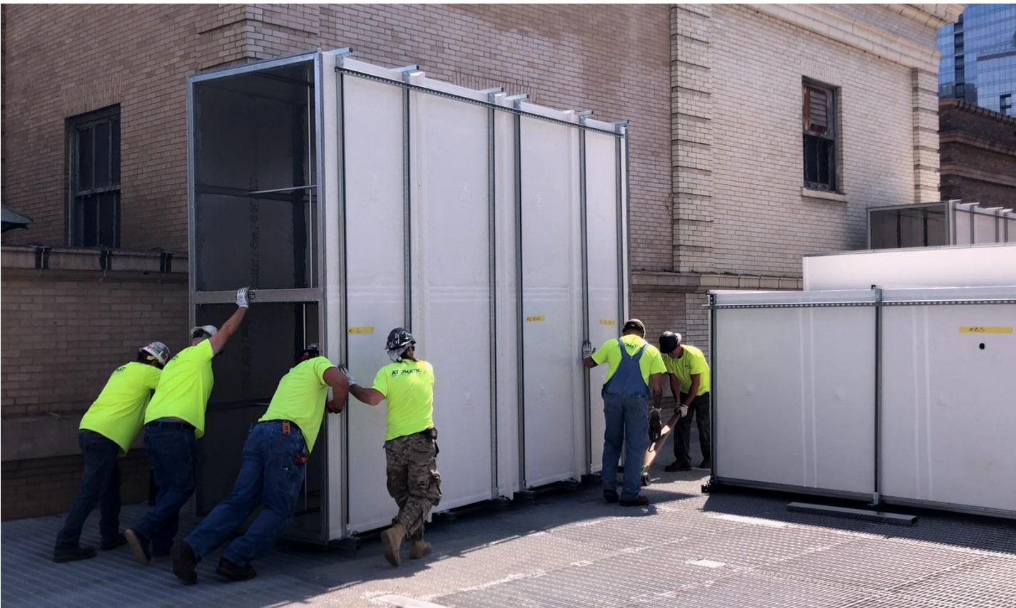
Transporting Thermaduct® across rooftop should utilize adequate methods to lift and not slide ductwork. Use necessary manpower to carry duct segments into place.
