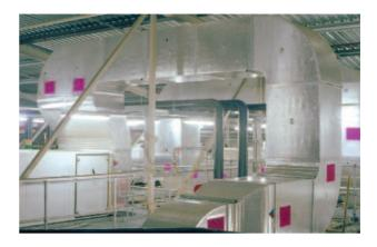
A key factor in the difference shown is in the cost of labor manhours. The construction, installation and insulation activity of the sheet steel ductwork system, accounted for 714.75 hours. In contrast, the fabrication and installation of ductwork from The *Kingspan* **Kool**Duct<sup>®</sup> System, only required 513.75 hours – providing a labor man–hour saving of 28%.
