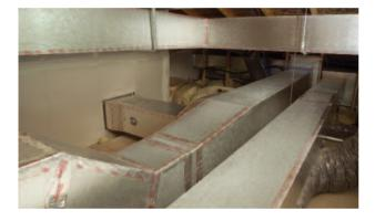
Traditionally, ductwork is constructed from galvanized sheet steel, which is installed first and then insulated separately as a second operation. The *Kingspan* **Kool**Duct<sup>®</sup> System however, is an advanced and innovative pre–insulated rectangular HVAC ductwork system, which is installed in a single–fix.
