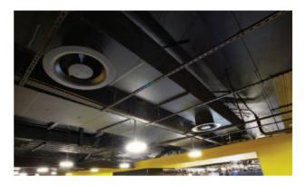
Ductwork fabricated from The *Kingspan* **Kool**Duct<sup>®</sup> System was the first premium performance pre-insulated ductwork in the world to be UL Listed as a Class 1 Air Duct, to Standard for Safety UL 181 (Underwriters Laboratories: Factory Made Air Ducts & Air Connectors), when fabricated to a specification clearly defined by UL.
