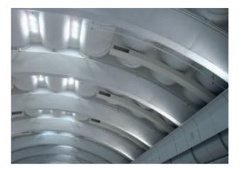
Kingspan Insulation commissioned a review by independent consultants, Rider Levett Bucknall, of the implications of reduced fan power on actual energy usage. Rider Levett Bucknall concluded that for a 328 ft / 100 m long run of ductwork, with cross–sectional internal dimensions of 24" x 24" / 600 x 600 mm and an air velocity of 1476 fpm / 7.5 m/s, ductwork fabricated from The *Kingspan* **KoolDuct®** System could save 10.5 MMBtu / 3100 kW·h per annum.
