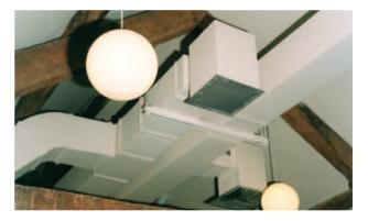
In addition, ductwork fabricated from The *Kingspan* **Kool**Duct<sup>®</sup> **System** can reduce air–leakage rates to a fraction of those typical of rectangular sheet metal ductwork. This cutting edge System thus offers the triple benefits of cutting energy use, cutting operational carbon dioxide (CO<sub>2</sub>) emissions and cutting costs.
