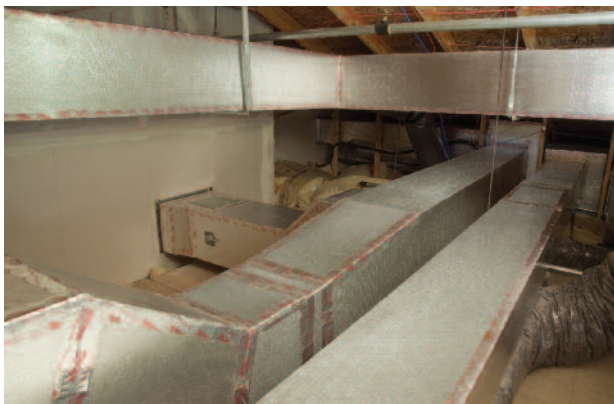
Figure 4: Cottage 6A, Kingspan KoolDuct ® System Ductwork Installation
