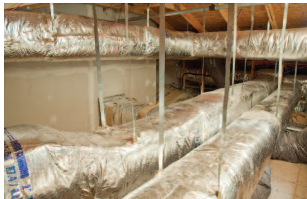
Figure 5: Cottage 6B, Glass Fiber Insulated Sheet Metal Ductwork Installation
