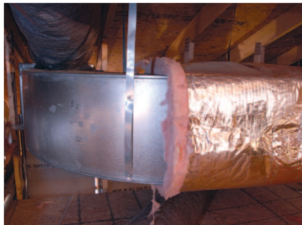
Figure 6: Sheet metal ductwork requires a separate manual wrapping operation
