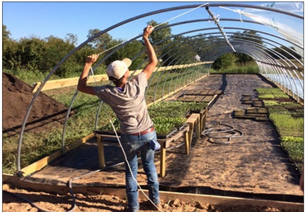
Building a hoop house at Farmshare Austin
