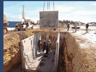
Constructing the Cellar
