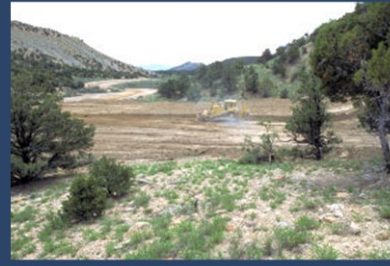
Excavating the Drill Site
