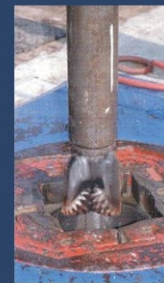
Lowering Drill Bit into Rotary Table
