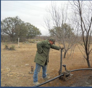
Repairing Flow Lines
