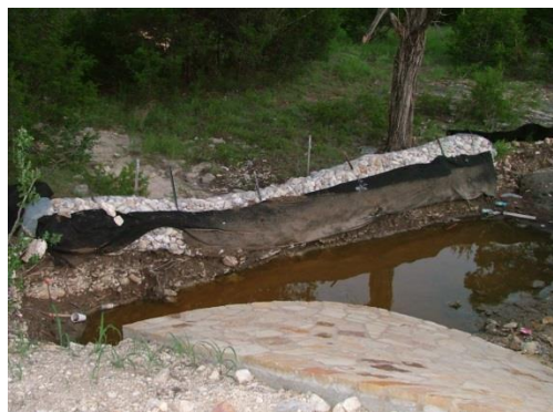
Temporary Gabion and Silt Fence
