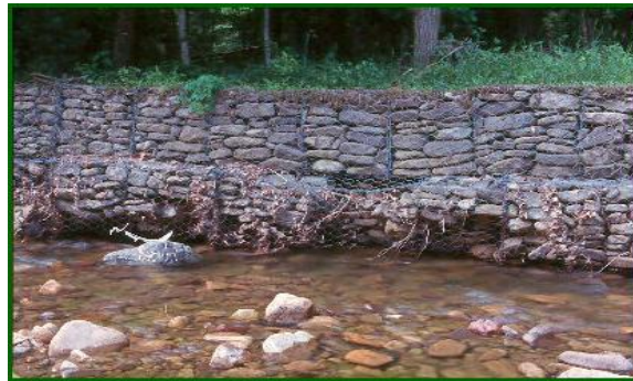
Permanent Gabion in creek bed
