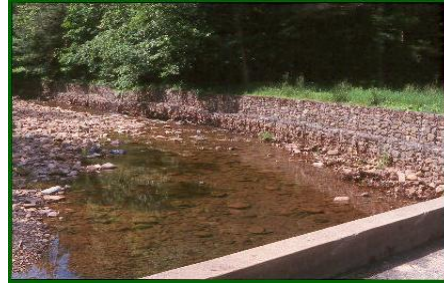
Permanent Gabion in Creek bed
