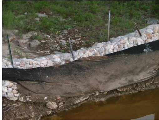
Temporary Gabion and Silt Fence
