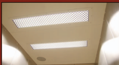
Fluorescent lights with polycarbonate diffuser panels flush mounted in canopy (Shown with optional vandal guard)
