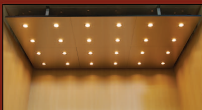
Low voltage mini down lights mounted in multi-panel drop ceiling
