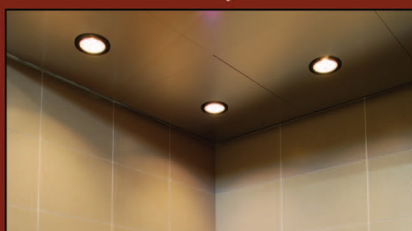
Incandescent down lights mounted in multi-panel drop ceiling
