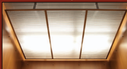
Fluorescent lights above aluminum frame with aluminum eggcrate diffuser panels
