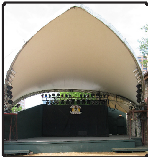
FRONT VIEW OF STAGE
