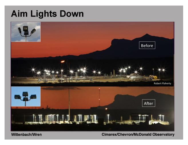
Construction and permanent lighting should be mounted and directed to focus light only on the intended area, and to avoid light spill and offsite light trespass. Lights pointing upward or horizontally should be avoided.
